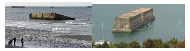
The Phoenix caisson was built in 1943-4 as a floatable breakwater component of the Mulberry Harbour which was considered to be a major technological and engineering achievement. It was effectively a mobile port facility, designed to sink or float as necessary, and was used by the Allies to land troops and arms at Normandy as part of Operation Overlord.
