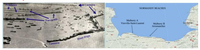
Phoenixes - 146 concrete caissons, 60 metres long, 18 metres high and 15 metres wide, making up **9.5 kilometres of** the breakwater.
